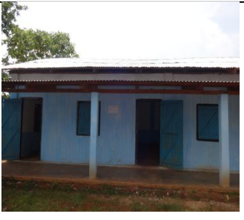
Building Front View
