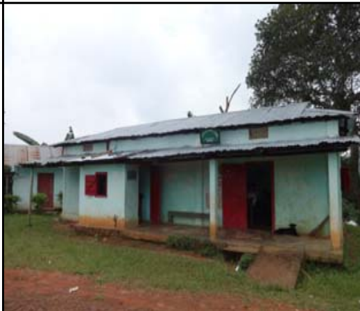
Building Front View
