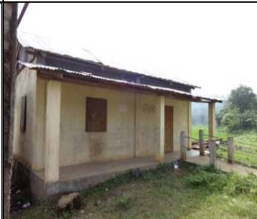
Building Front View
