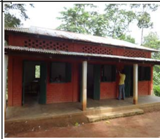
Building Front View
